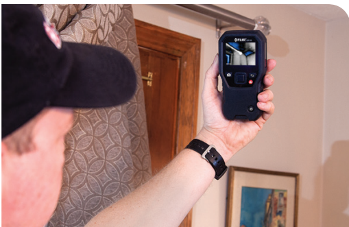
Scanning ceiling & wall joint for moisture issues
