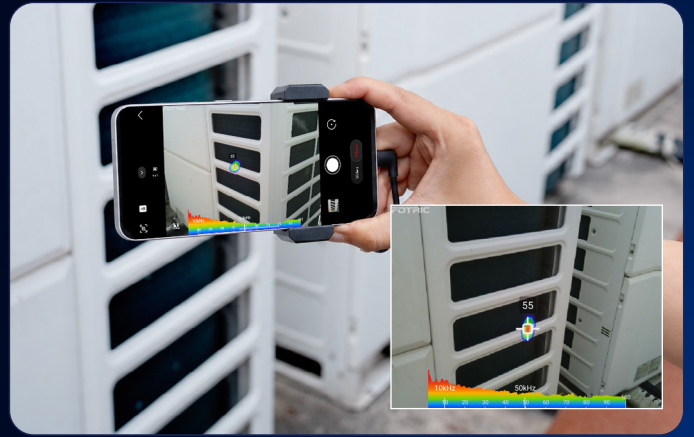
HVAC Air Leak Inspection
