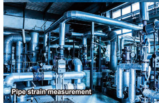
Brake and pipe strain measurement
