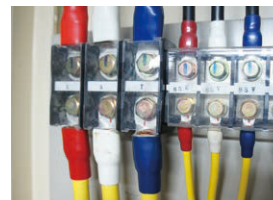
Locations with covered terminals
